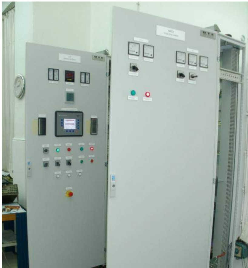
CHP, 400kVA on biomass Control cabinet
