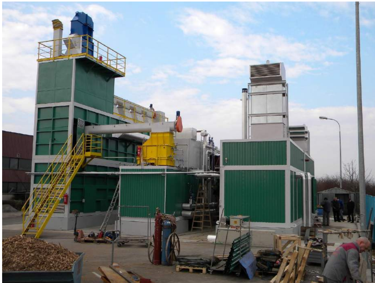
CHP, 400kVA on biomass
