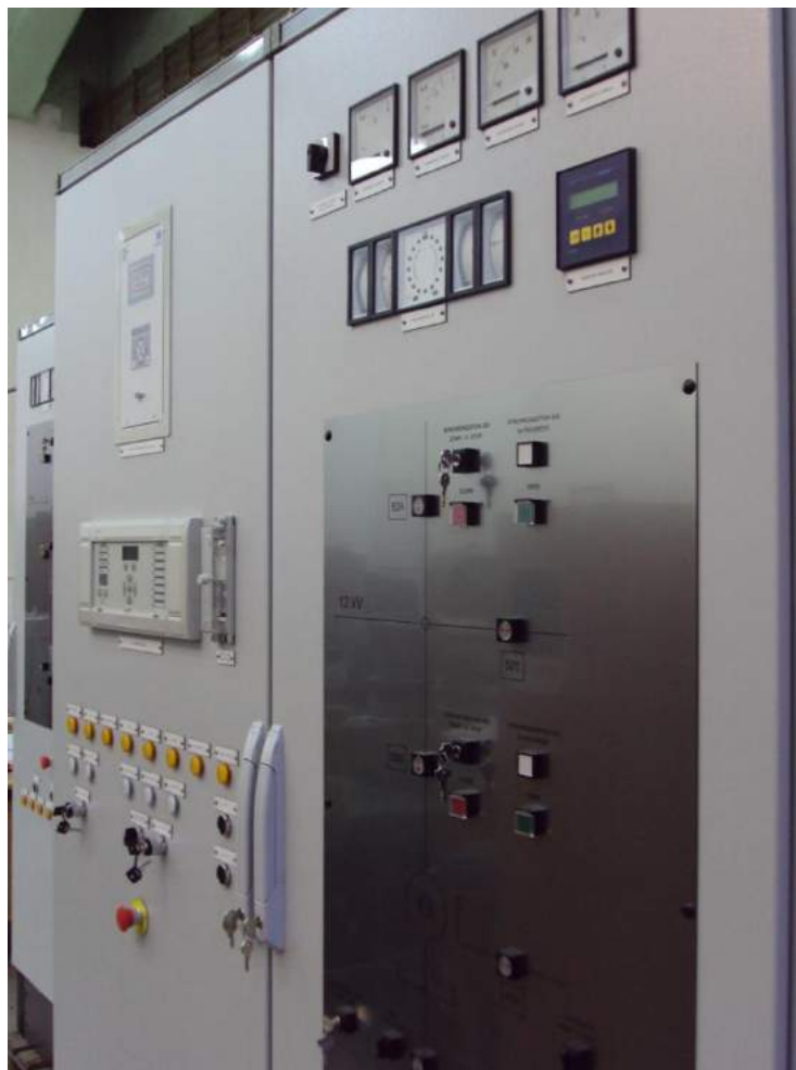
32,5MVA, 12kV generator excitation and protection cabinet Ta-Lin refinery, Taiwan
