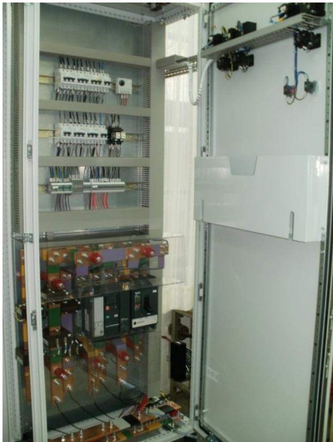
CHP, 400kVA on biomass Control cabinet
